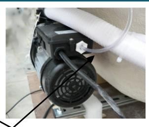
Check Capillary pipe is attached to on/off button and pump
